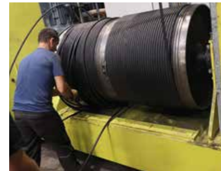
Dismantling the hoisting drum on the storage and retrieval machine
