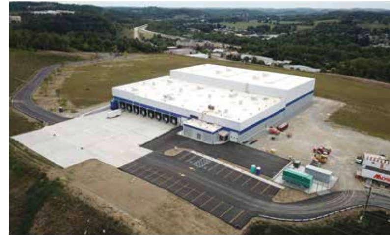
Ensinger's new building in Washington, PA
