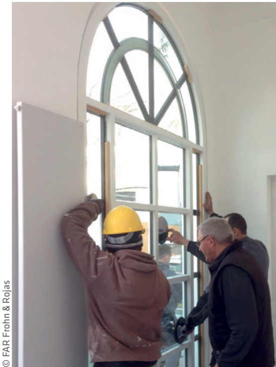
Installation of the new safety glass doors and windows.
