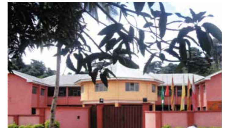
The construction of the school buildings was sponsored by donations
