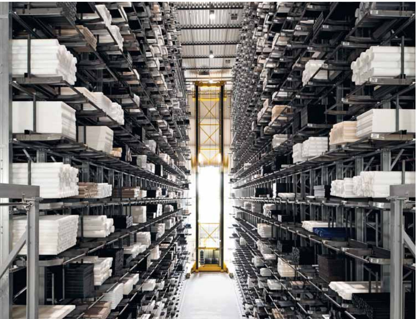
Glimpse into the high-bay warehouse: Rack handling device and stored stock shapes
