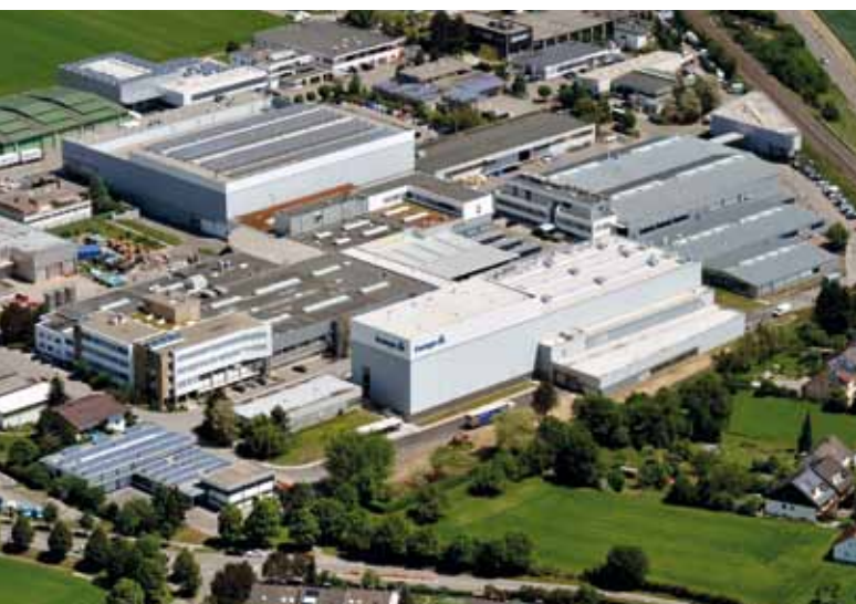
Ensinger's Nufringen location showing the new Stock Shapes Division building in the foreground
