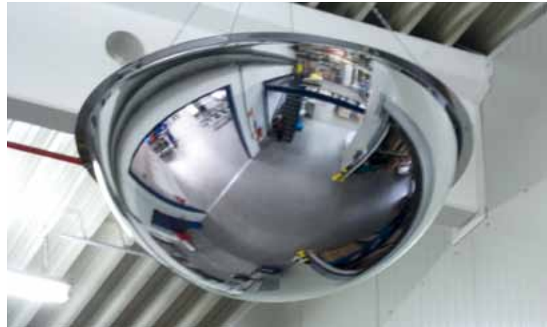
Another relatively simple solution for the prevention of accidents is to install round mirrors at poor visibility junctions. This is an effective way of preventing collisions between industrial trucks
