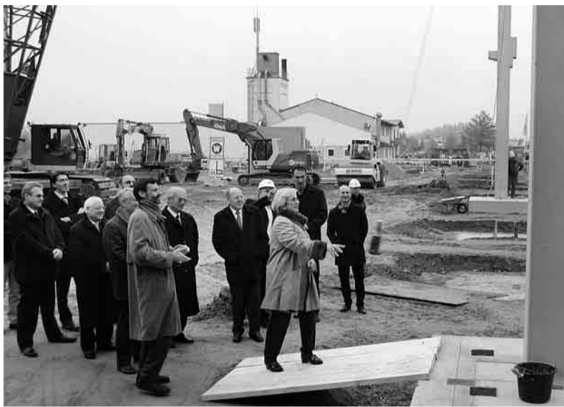
"Column christening" in Cham: Martha Ensinger gives the go-ahead for a new building project
